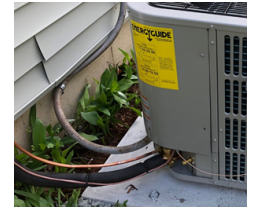
Install Linesets and Electrical
