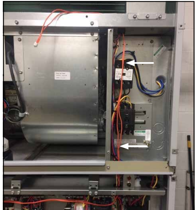
FIGURE 14 Route Orange Mixed Air Sensor Wires
