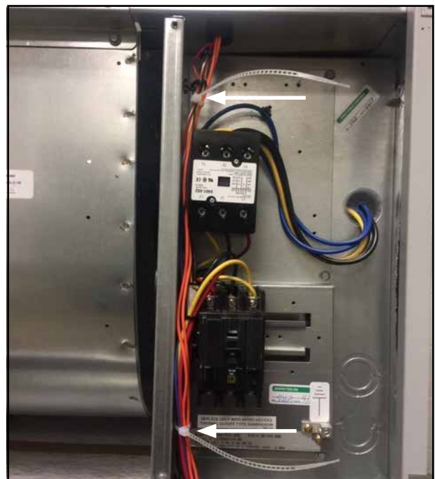
FIGURE 15 Secure Sensor Wires with Ladder Ties
