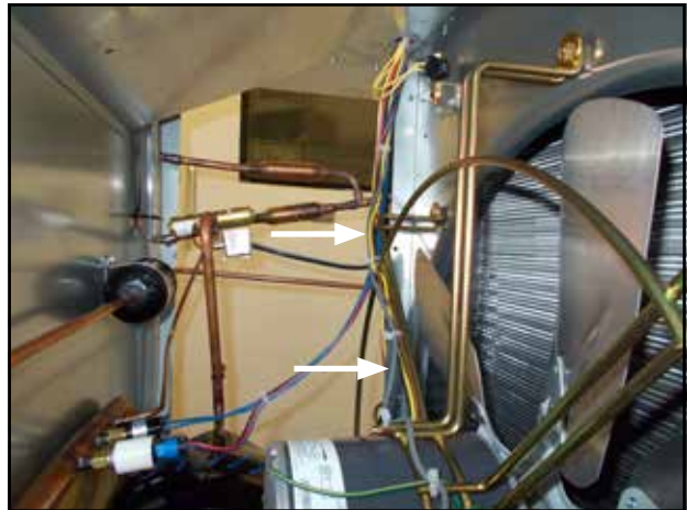
FIGURE 19 Route Wires and Secure with Ties
