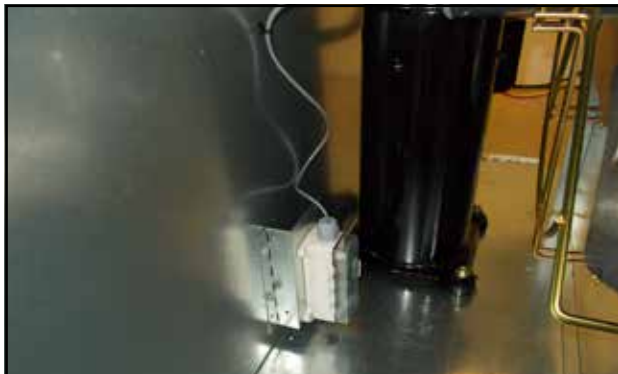
FIGURE 17 Enthalpy Sensor Assembly Installation
