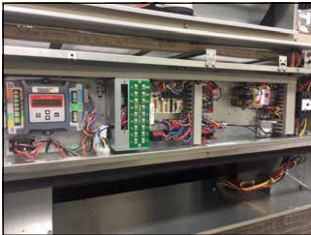
FIGURE 22 Wiring Connections Completed
