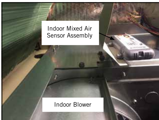
FIGURE 13 Install Indoor Mixed Air Sensor Assembly
