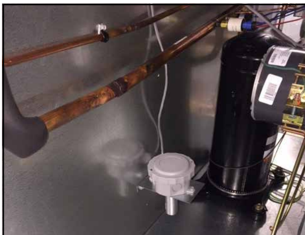
FIGURE 18 Temperature Only Sensor Assembly Installation
